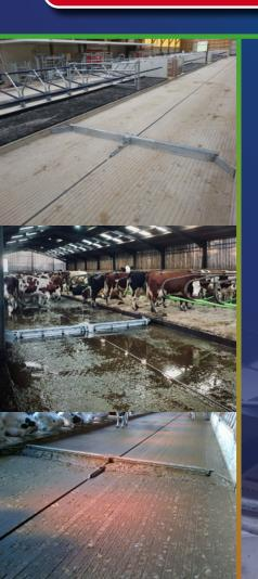
The Dairypower Eco-Clean Rope / Cable scraper system can be used to efficiently clean up to four passages with the same drive unit controlling all the scrapers.
